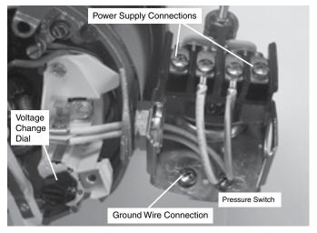
Figure 6: Voltage set to 230 volts, Dial Type
