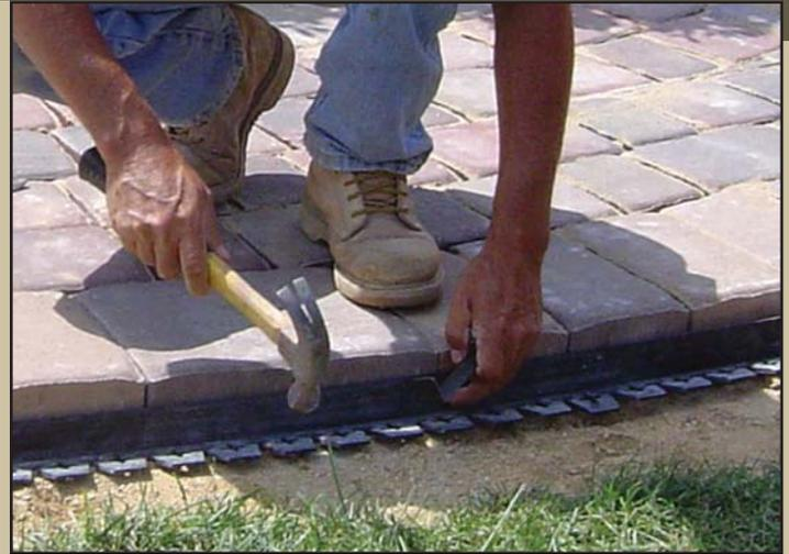
Slide the bottom section of Diamond-Lok up to the sidewall until the edging sidewall is flush with the pavers.
