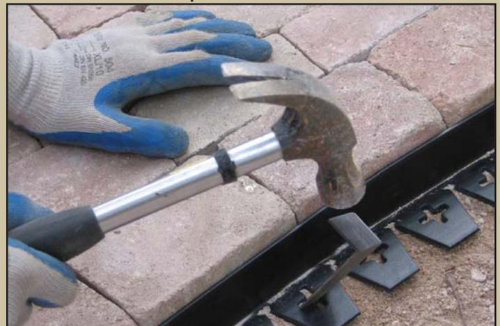
Anchor stakes need to be hammered in at a 45° angle with the head of the stake pointing up. (Always wear protective gloves and eye wear before striking anchor stake.)
