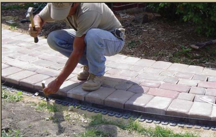
Install the stakes at each end and approximately every 2 feet by pounding them through the holes provided at a 45° angle facing the pavers.
