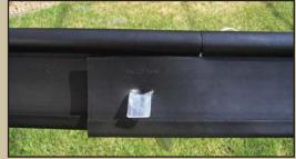
Drive an anchor stake through both sections of edging.
