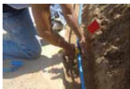
2. Cut-into the lateral line
