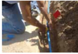
2. Cut-into the lateral line
