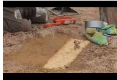
Mound Hole Repairs with Clay Blocks 1:17
