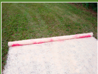
Figure 1. Locate red dye line near the end of the ECB.
