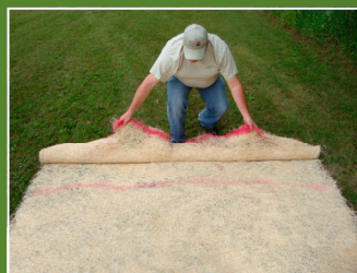
Figure 2. Pull end of ECB along red dye line.
