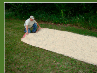
Figure 4. Properly position unrolled ECB for installation
