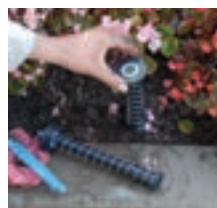
Remove the "guts" of Rain Bird 1806 spray head
